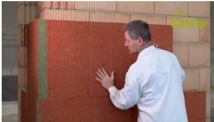
Workflow step: Placing the insulation board
